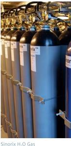
efficiently combines nitrogen with cooling water mist.
